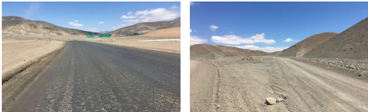
Figure 10: Non-Paved B-240 Road with Bischofite Covering (Left) and Road to Proposed Plant Site (Right)
