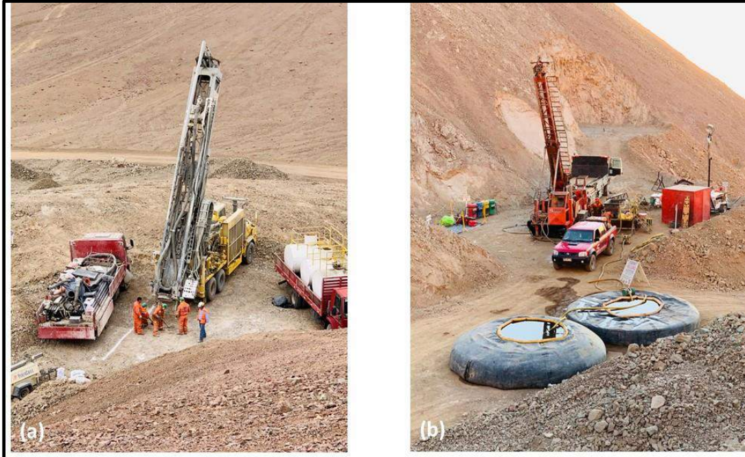
Figure 9-2: Photos from Drilling equipments (a) Reverse Air: (b) Diamond Drill
